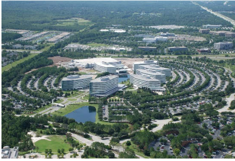
Blue Cross Blue Shield Florida Campus consisted of the design of the Power Distribution, Power/Lighting Design, and Fire Alarm Design.
