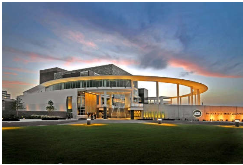
Long Center for the Performing Arts included MEP engineering with coordinating with specialist contractors such as the lighting specialists and audio and visual specialists.
